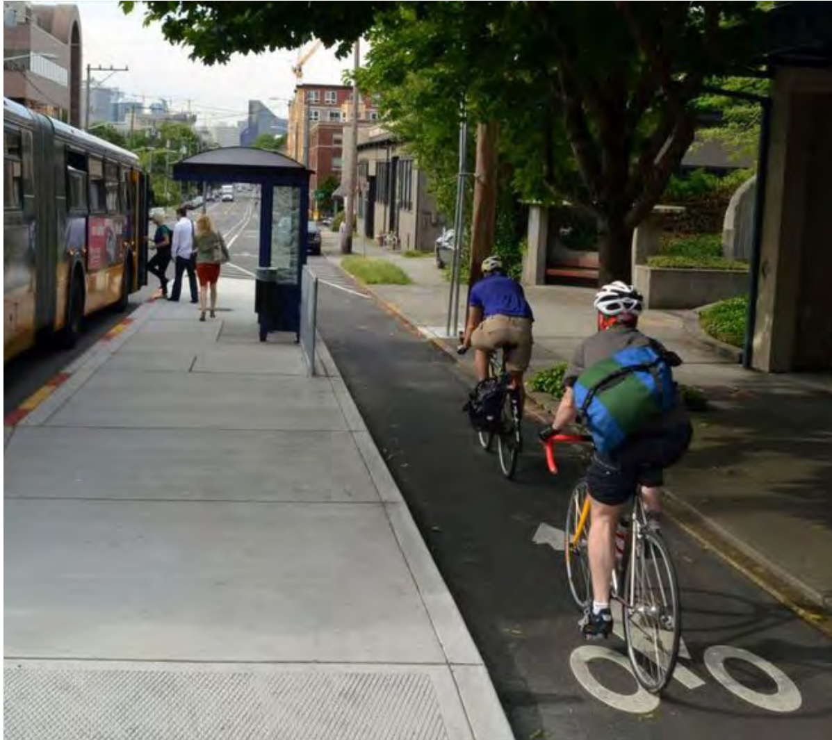
Figure 39. Floating bus stop
