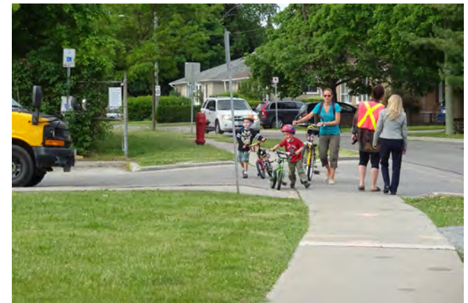
Figure 11. Sidewalk continued through driveway at Aurora Heights Public School in Aurora, ON
