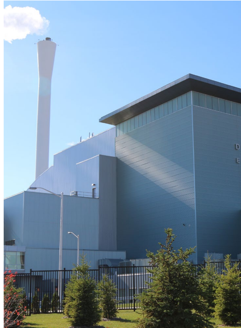
Durham-York Energy Centre
