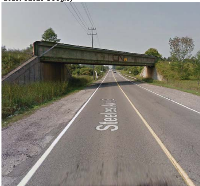
Railway underpass east of Ninth Line (Image capture: 2015, ©2016 Google)
