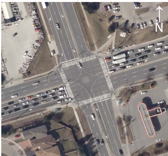
Steeles Avenue at Kennedy Road
