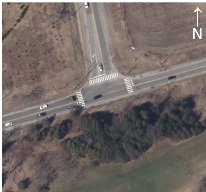
Steeles Avenue at Ninth Line
