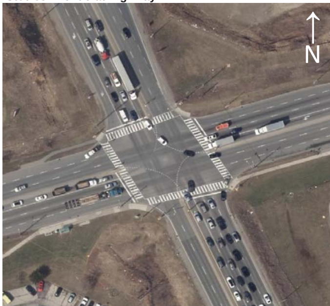
Steeles Avenue at Highway 27
