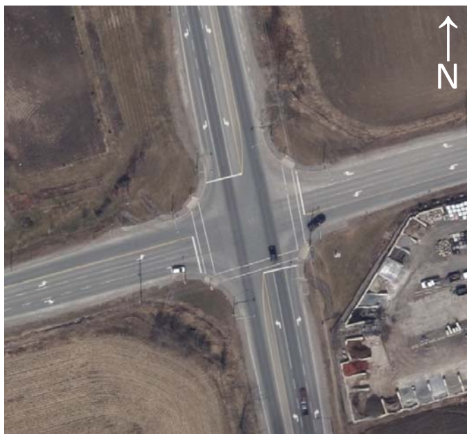
Woodbine Avenue at Old Homestead Road
